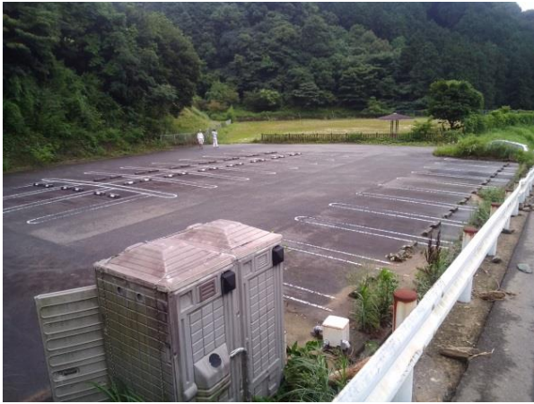
(仮置場開設前)
